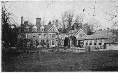
Enham Place and the New Medical Block.
