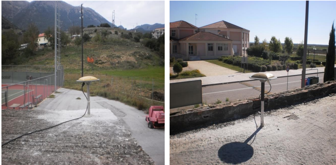
Figure 4-2. Photos of newly installed PaTrop GNSS permanent stations in Kalavrita (left) and Mesologgi (right)
