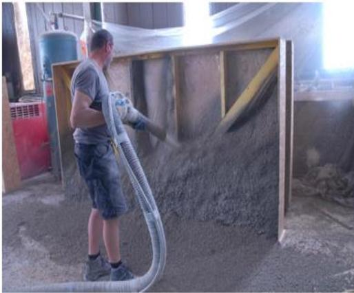
Figure 1. 37: Filling the timber frame with hemp.
