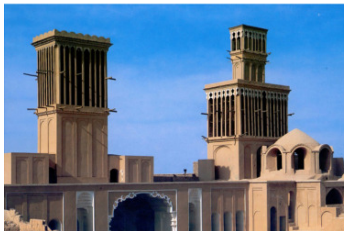
Figure 2.3: A two story wind tower along with the dome (Kolah-farangi) of the Aghazadeh mansion in Abarkuh city, Yazd, Iran (Dehghani-Sanij et al., 2015)
