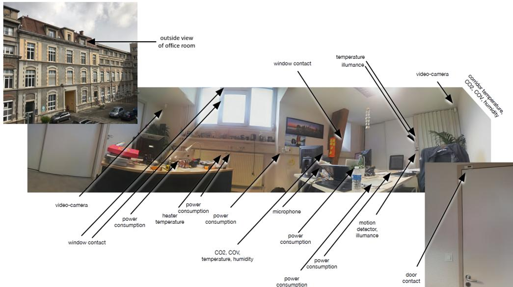
Figure 4.1: Office at Grenoble Institute of Technology fitted with 27 sensors
