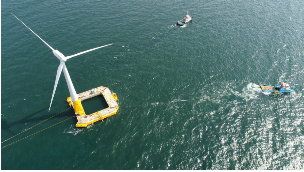
Figure 1.4 – Installation of the Floatgen wind turbine ©Centrale Nantes/ABOVE ALL.
