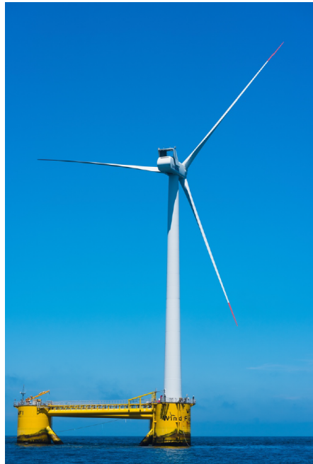
Figure 2.14 – Full-scale testing in the WindFloat project (from [Roddier et al., 2017])
