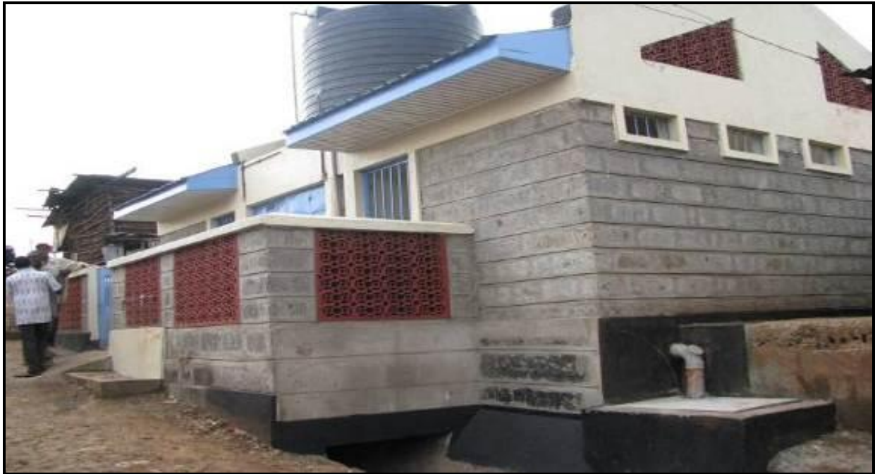
Plate 1. 9: A sanitation block in Soweto East
