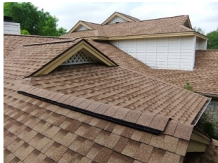
Roof shingle material (b)
