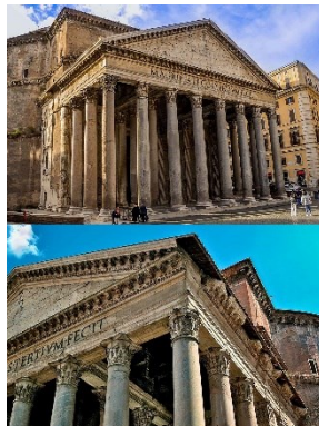
Structural and decorative element
