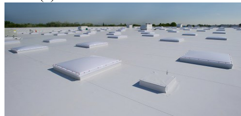
Roof membrane material (f)
