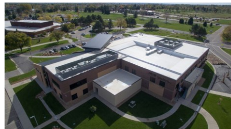
Flat roof (b)
