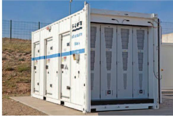
Figure 2.5: Picture of the installed lithium-ion battery of 1 MW / 560 kWh of SAFT [14].
