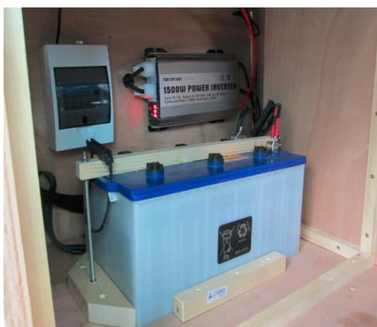
Figure 41 Power supply for the set-up (battery and inverter)
