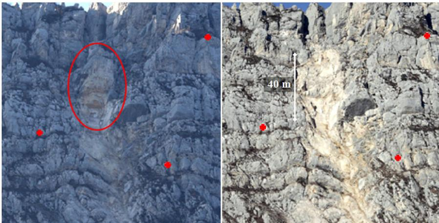
**Figure 2.3:** Unstable rock block before the blast (left); after the blast (right). Red crosses correspond to the control points used for georeferencing
