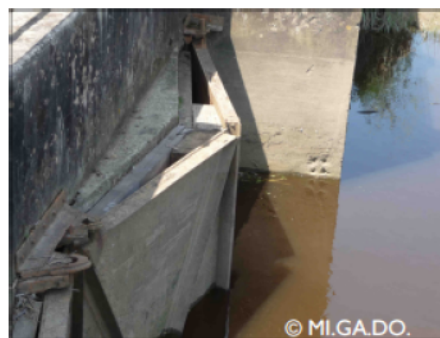
FIGURE 4.15: Cales portes (Source : MIGADO, 2008b)
