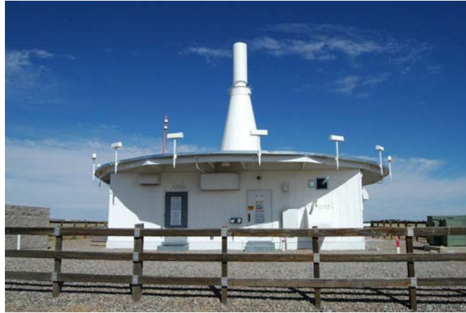
FIGURE B.1: VHF Omnidirectional Range ground station 4
