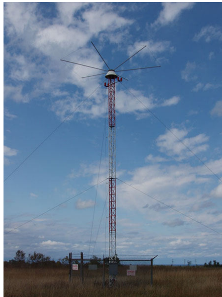
FIGURE B.2: Non-Directional Beacon 6
