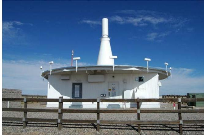
FIGURE B.1: VHF Omnidirectional Range ground station<sup>4</sup>
