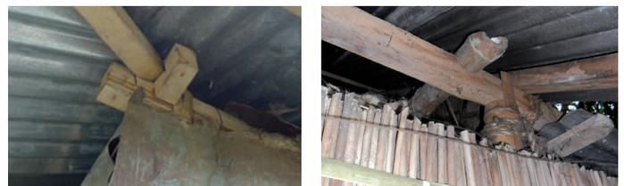
On the top of bamboo posts a special carving is used for better fixing of the beam. Special carvings are also done for bamboo beams and wooden posts connection.
