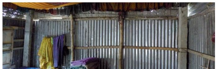
Mixed structure: concrete posts for the main structure and bamboo and/or wooden posts for the secondary structure
