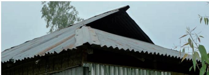
4 slopes roof: ridge piece with pointed shape to break the wind flow
