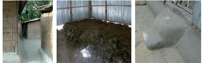
The plinth has a convex shape to facilitate the setting of the mud mixture creating a sacrificial mass
