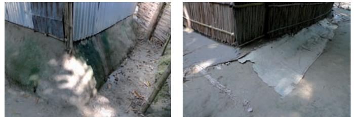
Degradation caused by water erosion, insects, and lack of maintenance
