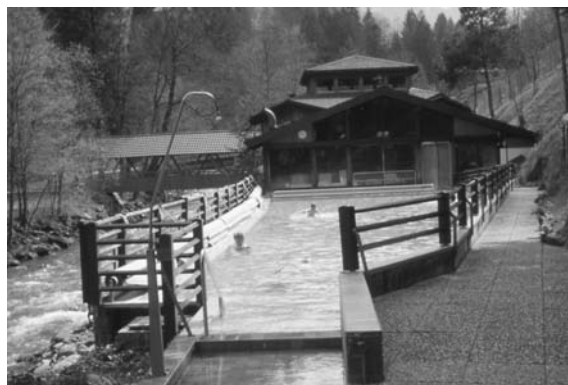
Figure 12.2: View of the Val d'Illicz spa (photo : H Rickenbacher, 1998)
