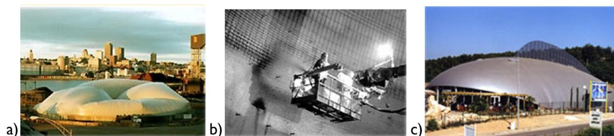
**Fig. 2.51:** a) Inflation of formwork; b) shotcreteing on the inside of the membrane; c) irregular shape structure constructed with pneumatic formwork [Pirs SA.]
