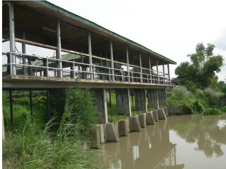
Figure 6-22 - Vanne de Sulipan (Macabebe).
