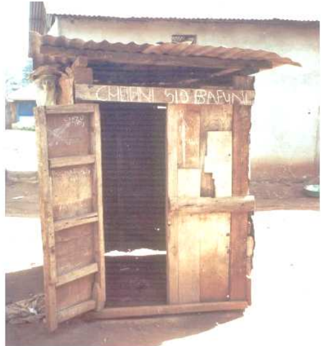
Latrines bas standing
