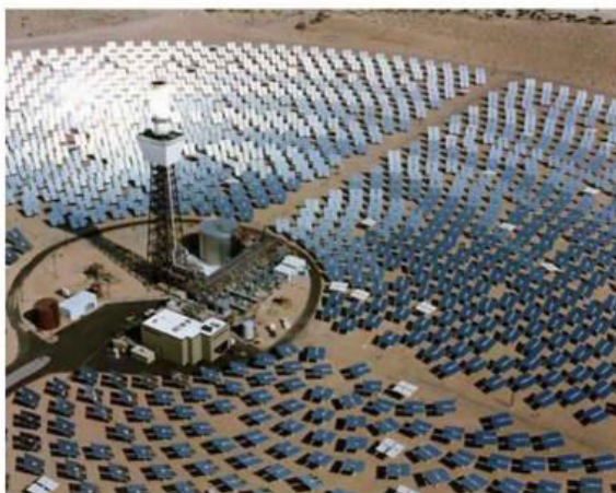
Figure 1-7 System and external receiver utilized at solar one facility in Barstow, California, USA [9, 10]
