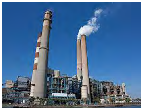
Figure 4.45: Example of power plant.
