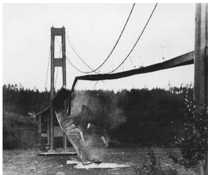
(a) Collapse of Tacoma Narrows Bridge (1940).
