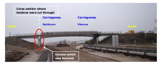
Figure 9.1 - S101 Bridge during damage test [VCE09].
