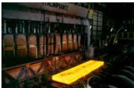
Walking beam reheating furnace
