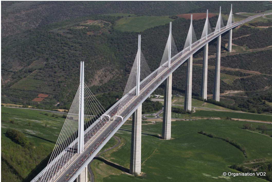
(a) General view of Millau viaduct.
