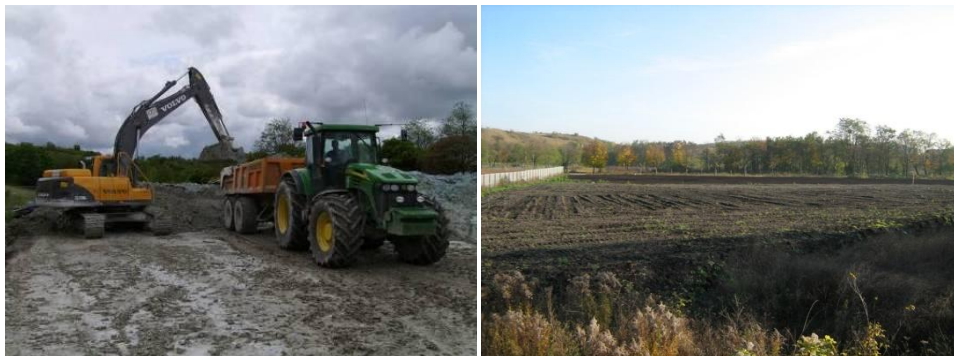
Fig. 2.1. Technosols during and after construction
