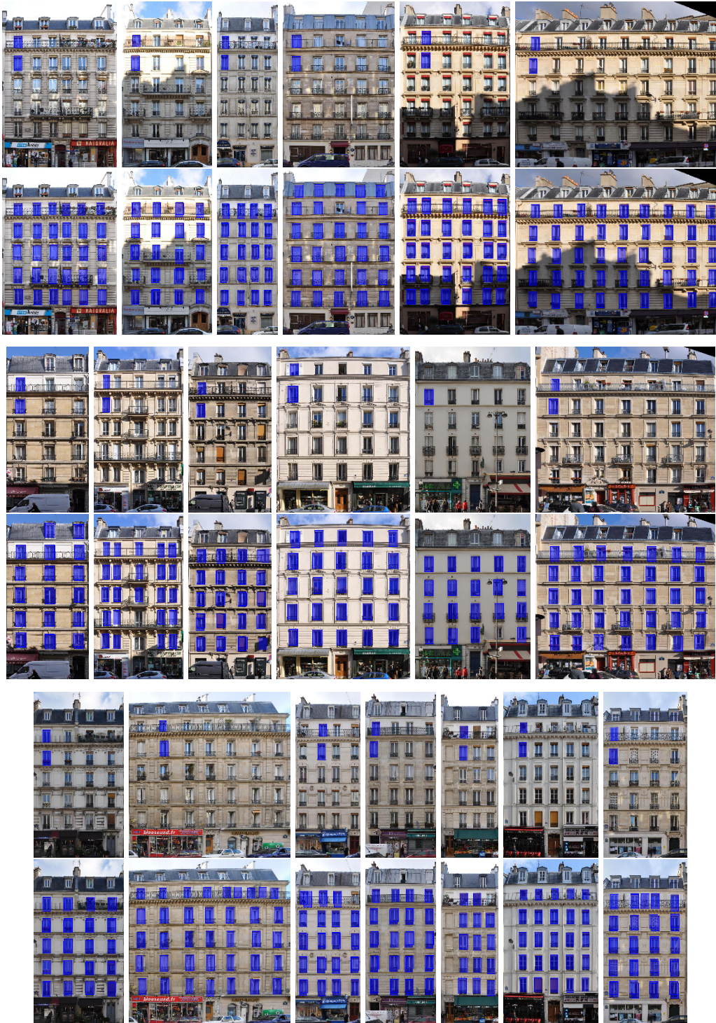
Figure E.4: Window detection results on the ECP Benchmark 2011 dataset. The odd rows show the input quadrilaterals and the even rows show the window detection results. (2/2)
