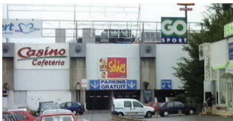
Figure 26 : Façade de Grand'Place Grenoble. Parking Nord
