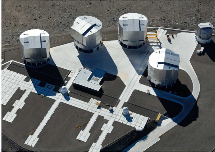
Figure 2.1: The Very Large Telescope. Are visible: the four unit telescopes (UTs) (from left to right: Antu, Kueyen, Melipal and Yepun), two auxiliary telescopes (ATs), the AT tracks and the VST (top left). Credits: ESO 1
