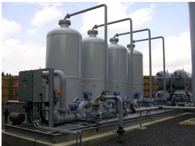
Fig. 5. Molecular Gate™ adsorption system for nitrogen and/or carbon dioxide removal (courtesy of Guild Associates, www.moleculargate.com ).
