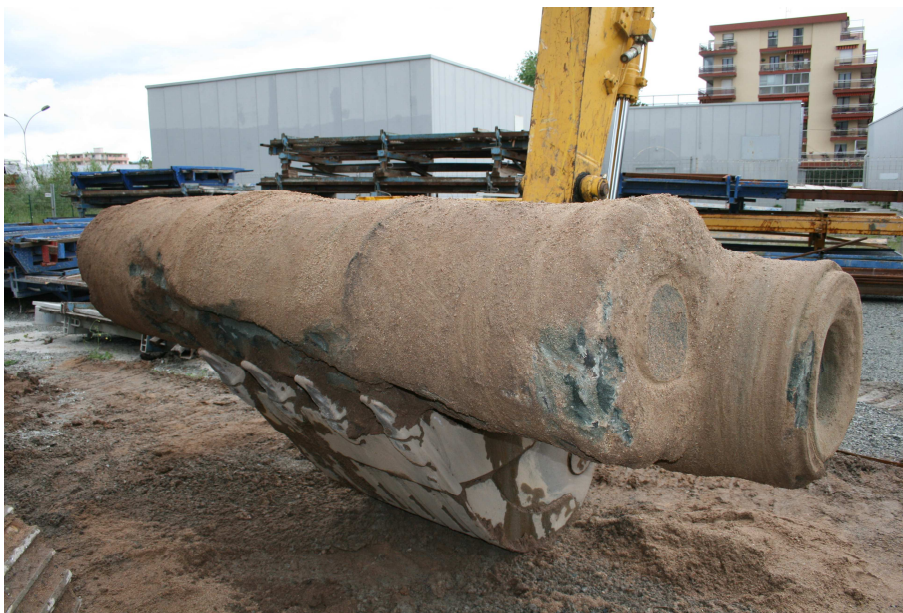
Figure 99 Colonne C3 excavée
