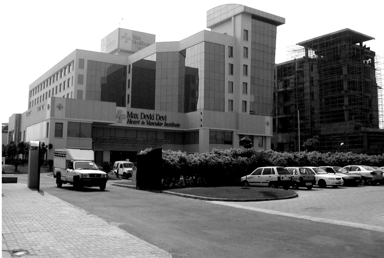
Illustration 21: Le Max Devki Devi Hospital et le Max Superspeciality Hospital en construction (2005)
