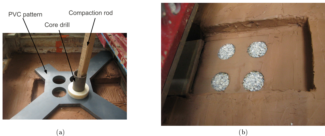
Figure 3.27: Installation procedure of the Load Transfer Columns surrounded by clay
