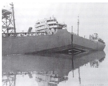
Figure 1.2 – The Schenectady tanker having its hull cracked almost in half while in harbor (1944).
