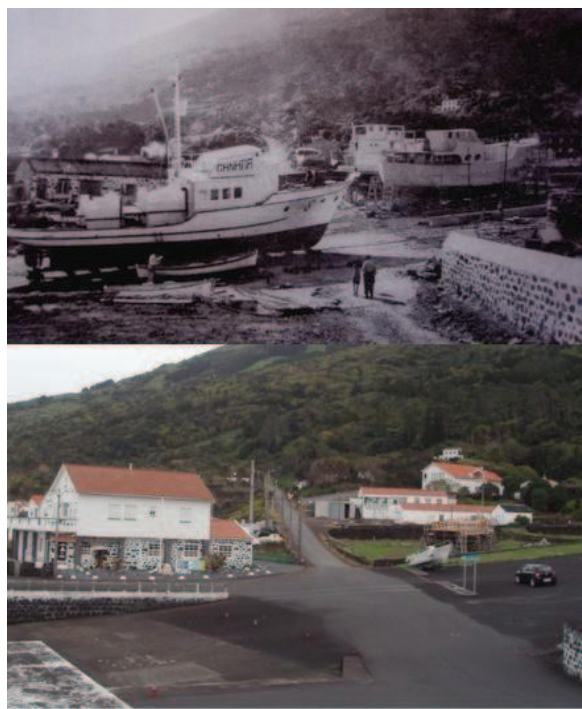
Figure 91 Chantier naval de Santa Amaro 1965 / 2009 - Pico.
