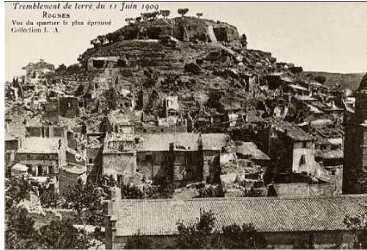
Figure 1.3: The Rognes hill after the Lambesc earthquake (1909, France). The effects of amplification induced by the presence of the hill are clearly visible in this picture taken few time after the ground motion.
