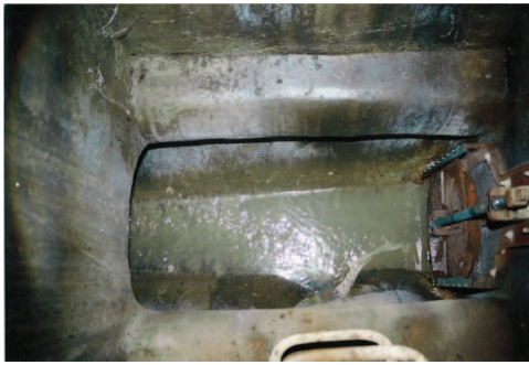
Figure 5.2.5.: Left: Picture of stormwater overflow device in the Chaudanne catchment (Pascal Breil). The overflow is regulated by a sewer port. Right: Spatial configuration for use of TDSO module. Ss means sewer system.
