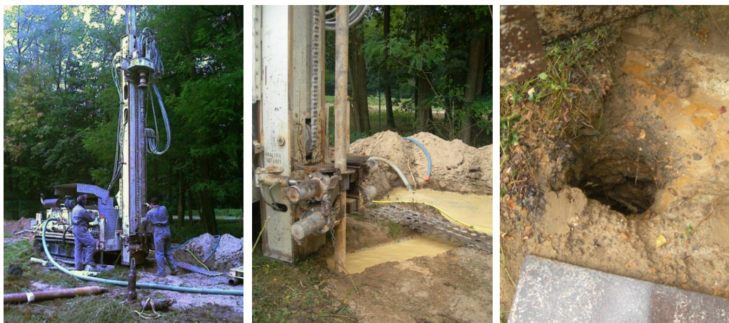
Figure 4.4: Drilling operation and borehole
