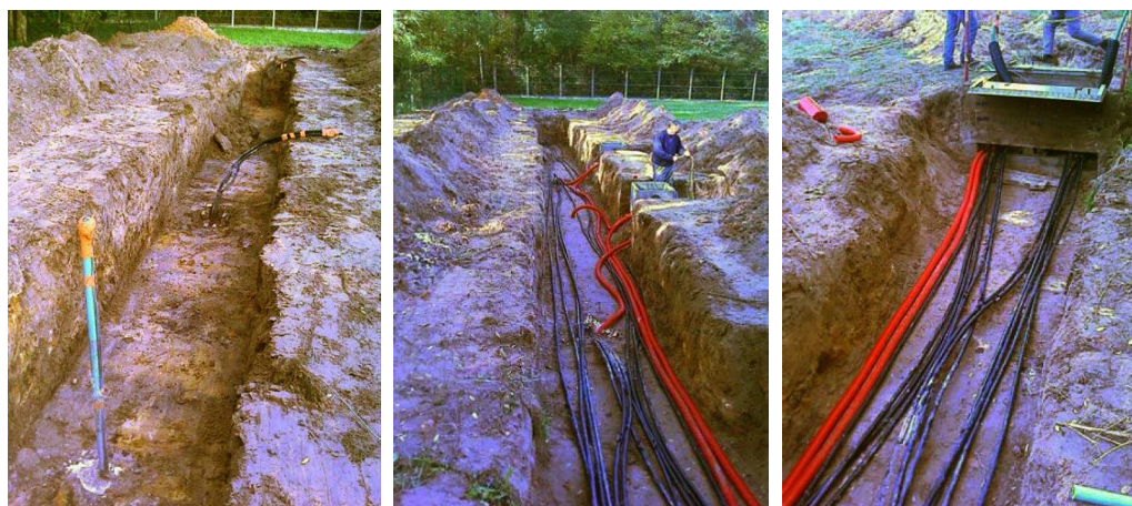
Figure 4.7: Sensor cable cutting and connecting to the manifold well (here, red pipes contain the sensor cables)
