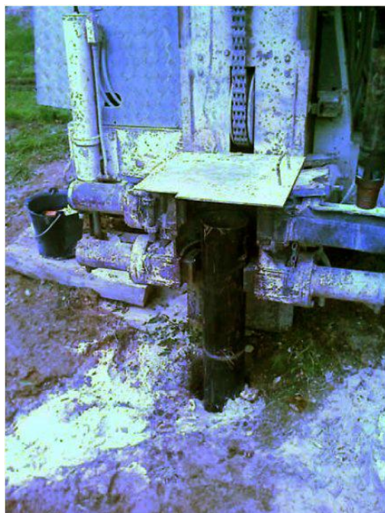
Figure 4.5: Case inserting
