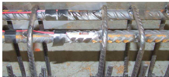
Figure 3.35 Strain gauges attached to the steel bars at mid span.*
