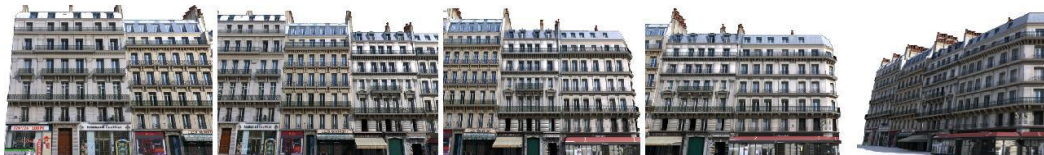
Figure 5.9: Urban dataset: the input dataset is composed of a set of calibrated photographs (pixel image resolution 1920x1080) and a coarse 3D model of the observed Parisian buildings.
