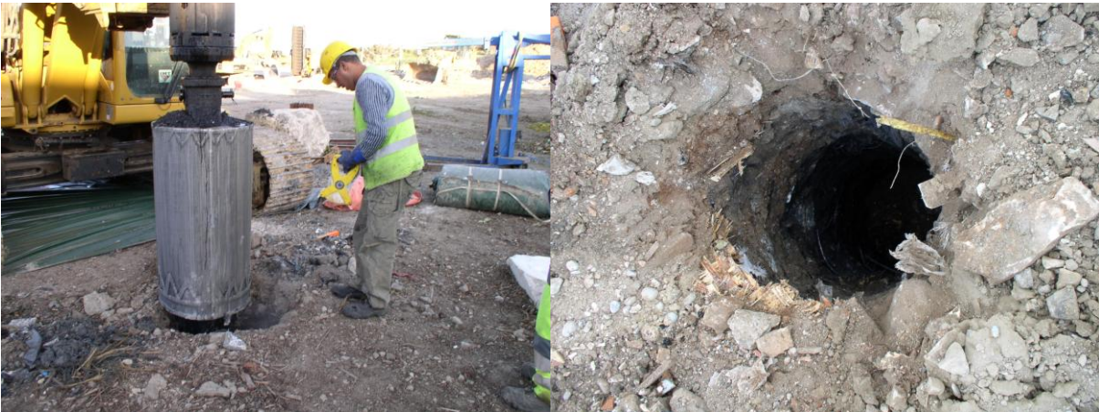
Figure VI- 42: Waste extraction at landfill site ‘N’.
