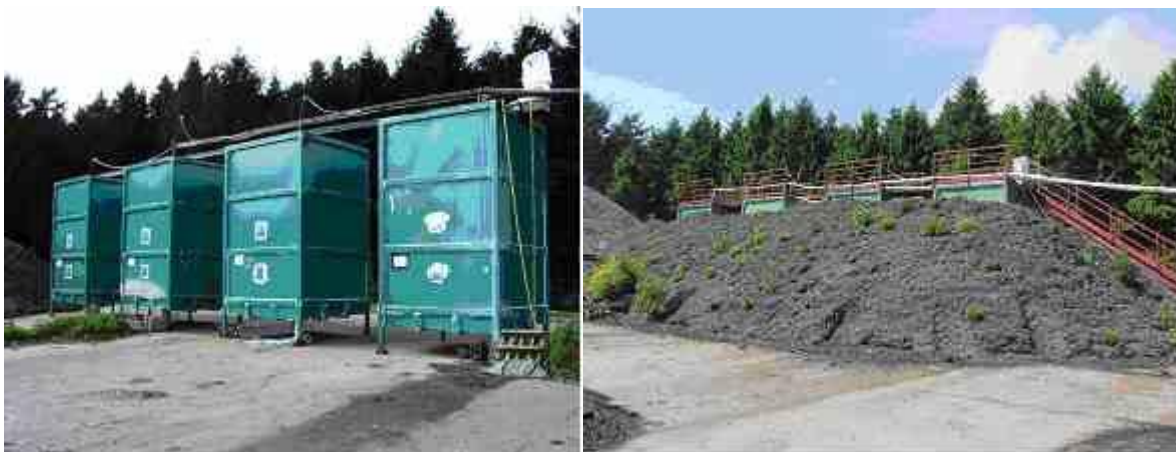
Figure III- 5: Study Cells of ELIA before and after the placement of cover compost.
