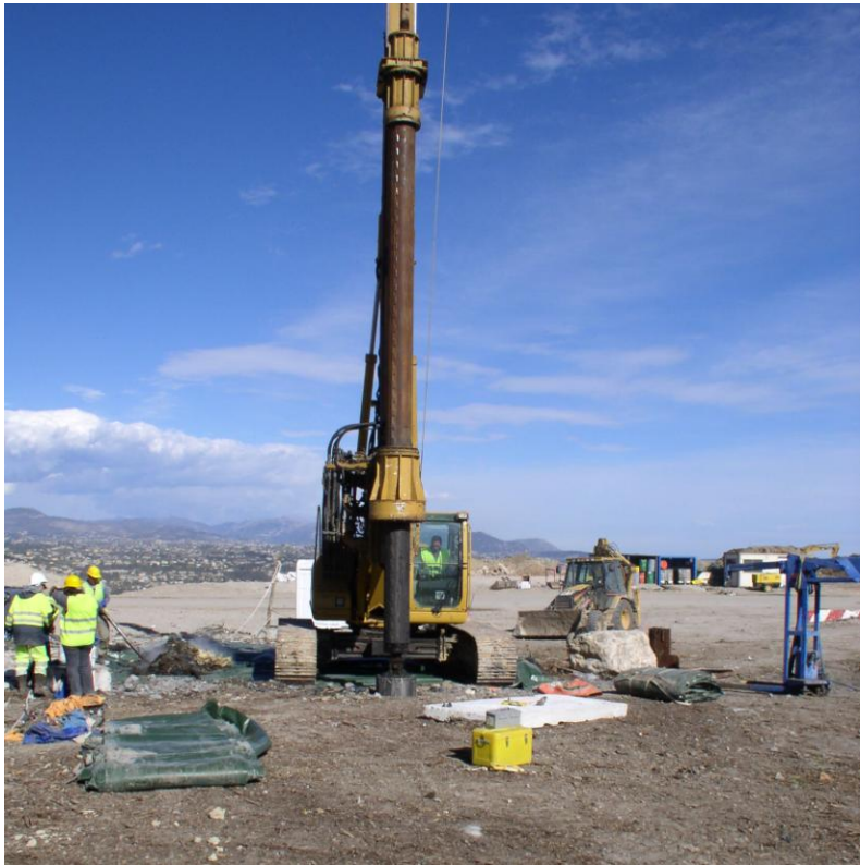
Figure VI- 40: Drilling operation at site.
