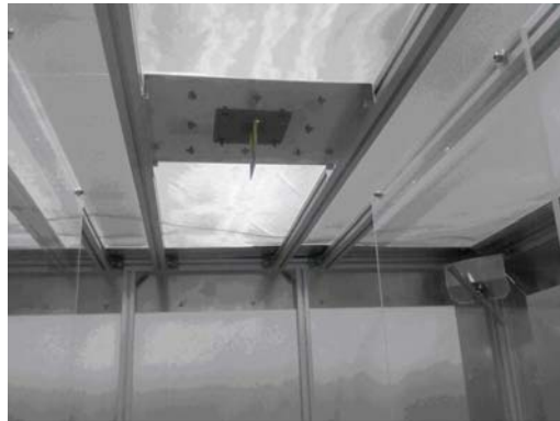
Figure 5.11 Realization and installation of the antenna in cavity
