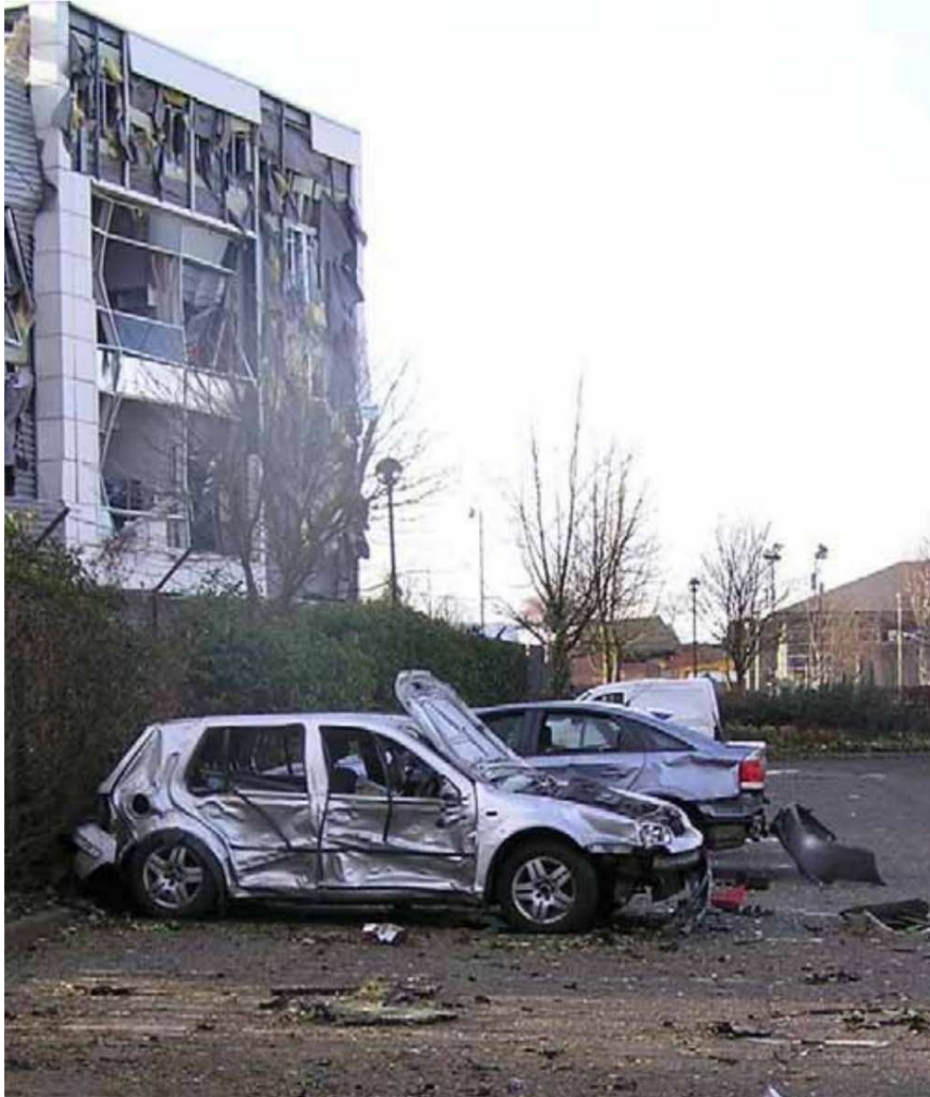
Figure 2: Photograph of damaged cars and buildings near the Buncefield depot taken approximately 400 meters from the main explosion site. This photograph is taken from Buncefield 2008.
