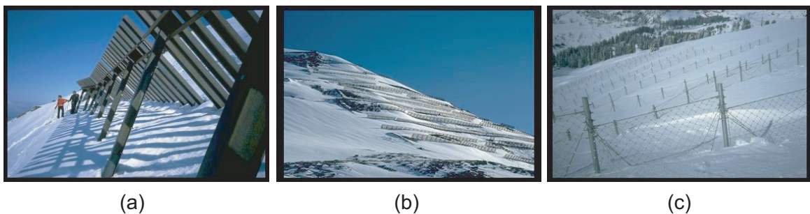
FIGURE 1.11: Divers types de protection active permanente. (a) Claies (photo F. Valla). (b) Rateliers et (c) Filets (photos F. Rapin).
