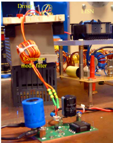
Figure 3.20: View of DC-DC boost converter, driver and LISN
