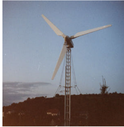
Figure I.5 : Eolienne de 10 kW [I.10]
