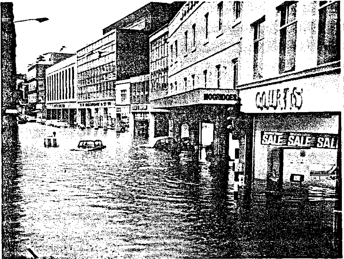
Flooding of commercial area (Reproduced by permission The Herald Express , Torquay).
