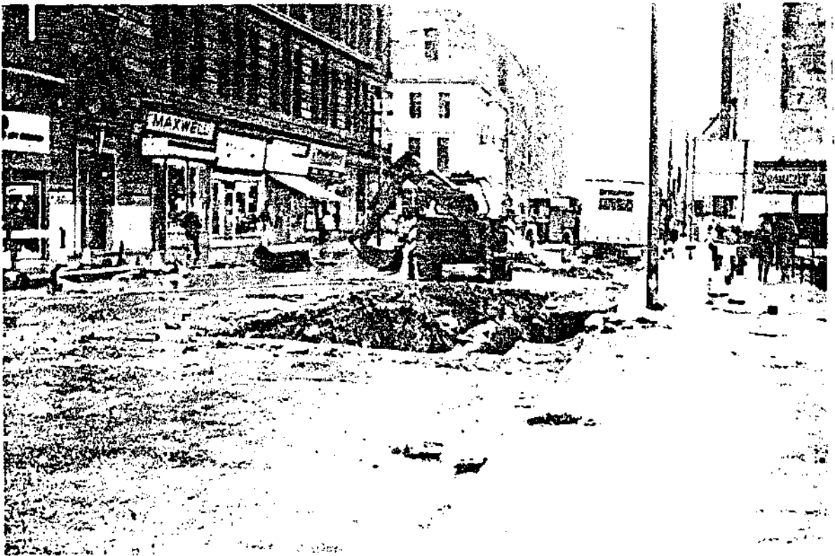
Collapse in commercial area (Glasgow).
