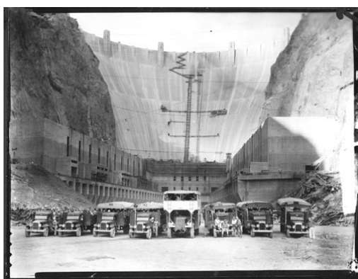
Figure 16 : Boulder Dam en construction.
