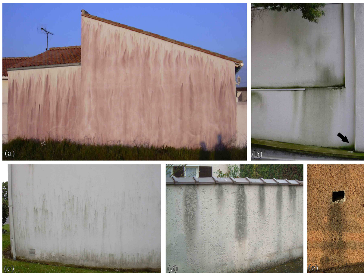
Figure 2. Some of the biofilms collected: (a) extensive red colonization by Trentepohlia iolithus on one-coat rendering mortar, along the Atlantic coast; (b) highly diversified green biofilm of algae and cyanobacteria developing on an organic finish beneath vegetation, and phenomenon of micro-humidity on the base of the wall, favouring extensive colonization (arrow); (c) green stains, dominated by Chlorosarcinopsis minor , developing on paint; (d-e) black stains, composed of algae and cyanobacteria, appearing in zones of high micro-humidity, beneath joints of tiles (d) or beneath an evacuation of balcony (e).
