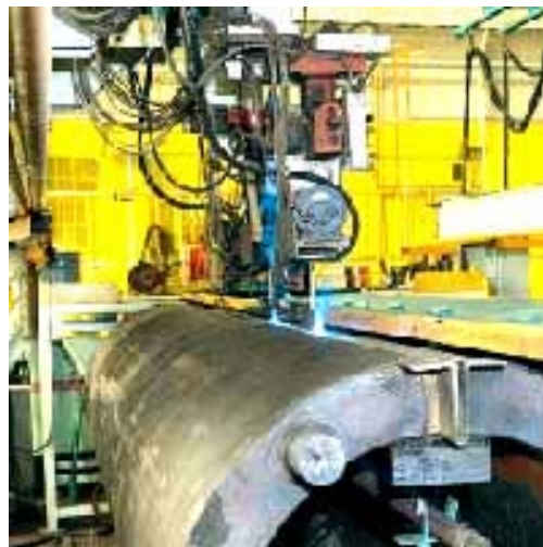
Figure In.3. Example of the welding operation on a pipe (source www.altavista.com )
